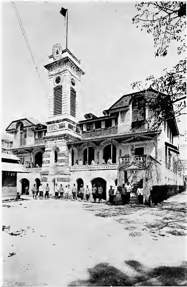
CENTRAL POST OFFICE
